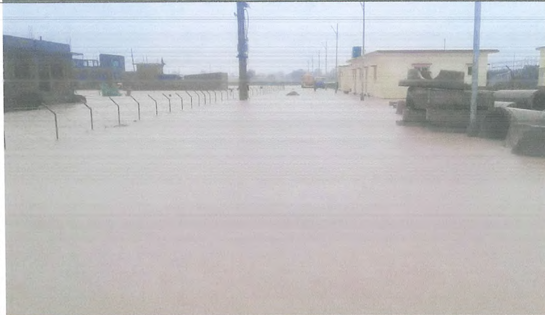
Water entered into lab building; ding inside STP behind the fence with wall is MD1
