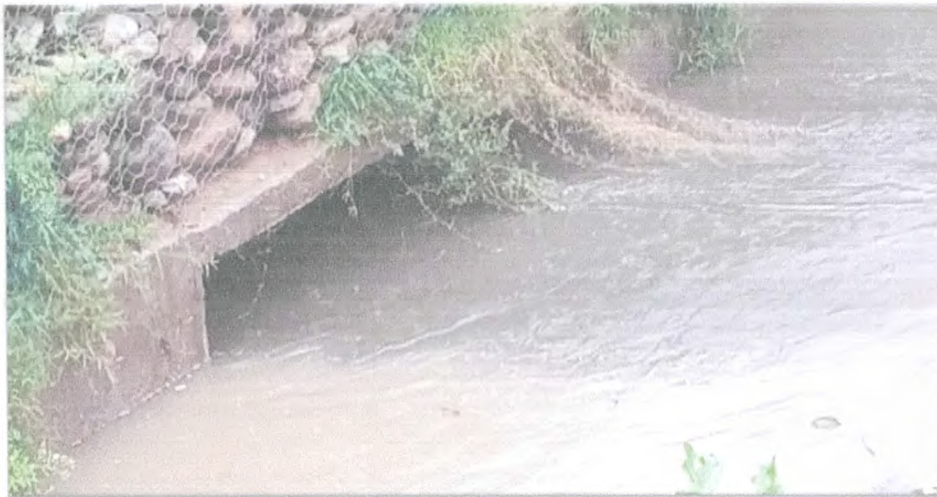
Stage-3 of Overtopping and Plugging of Outfall-9 during rainfall
