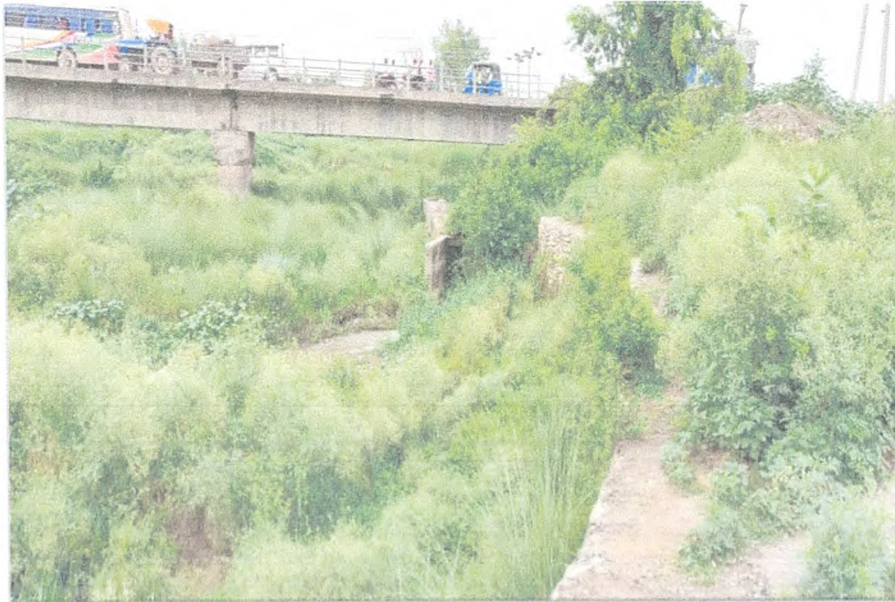
Sirsiya River Outfall-9 (size=2.60x1.80)m.
