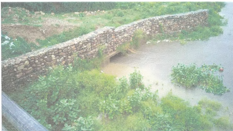
Stage-3 of Overtopping and Plugging of Outfall-9 during rainfall
