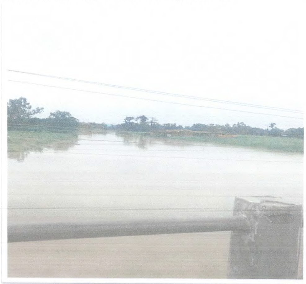
Stage-7 Sirsiya River bridge submerged due to high flood level.
