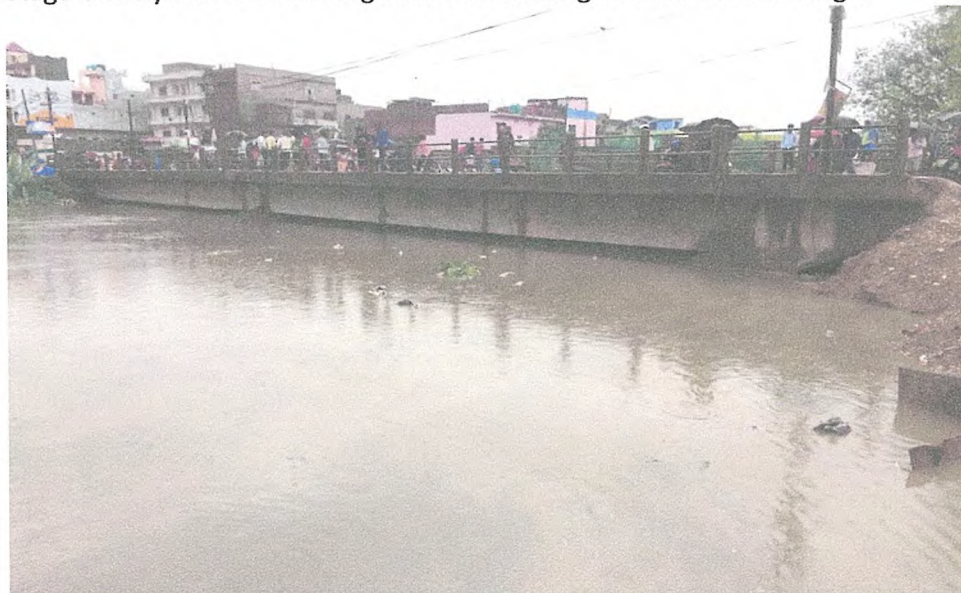
Stage-6 Sirsiya River course high flood level rising to deck level of bridge.
